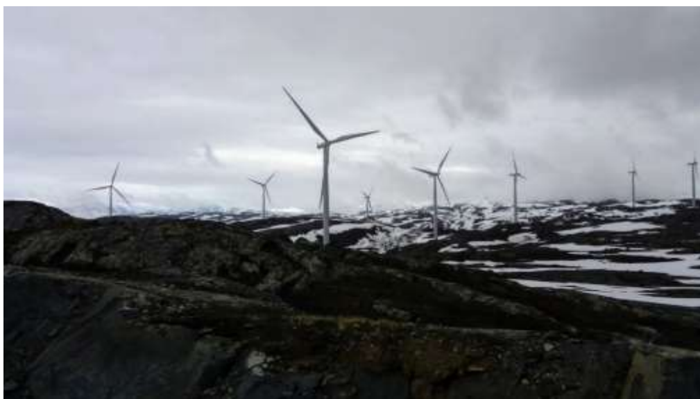
Figure: Fortum Nygårdsfjellet wind farm operated by Nordkraft.
