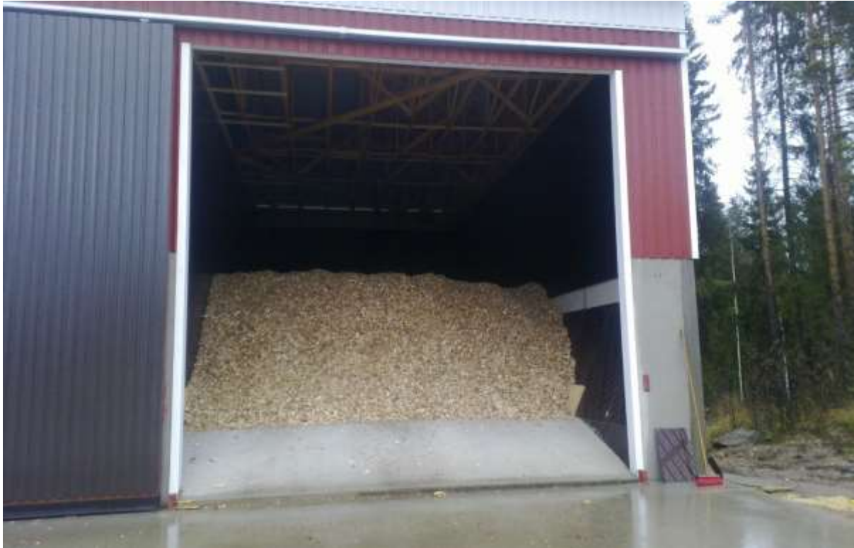
Figure 2. Woodchip dryer and storage 2
