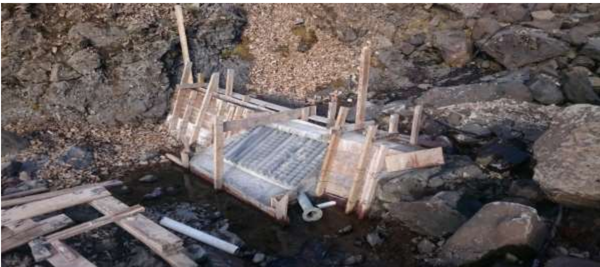
Figure 5 The box installed into the stream. 5
