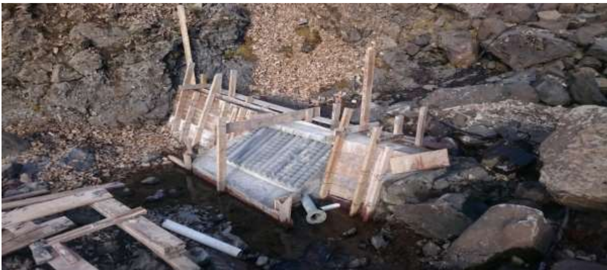
Figure 5 The box installed into the stream. 5
