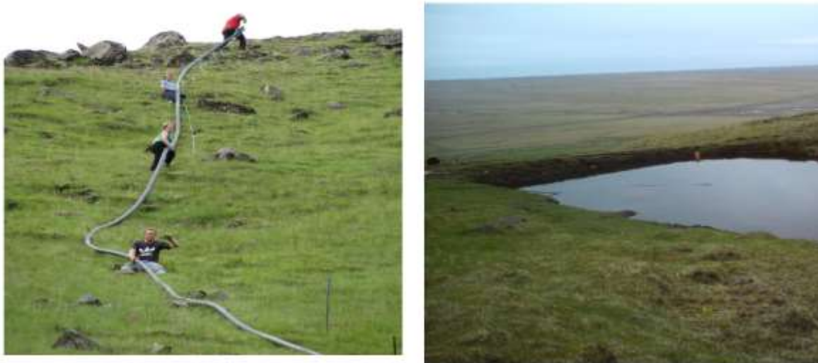
Manpower used to construct the pipeline from the stream
